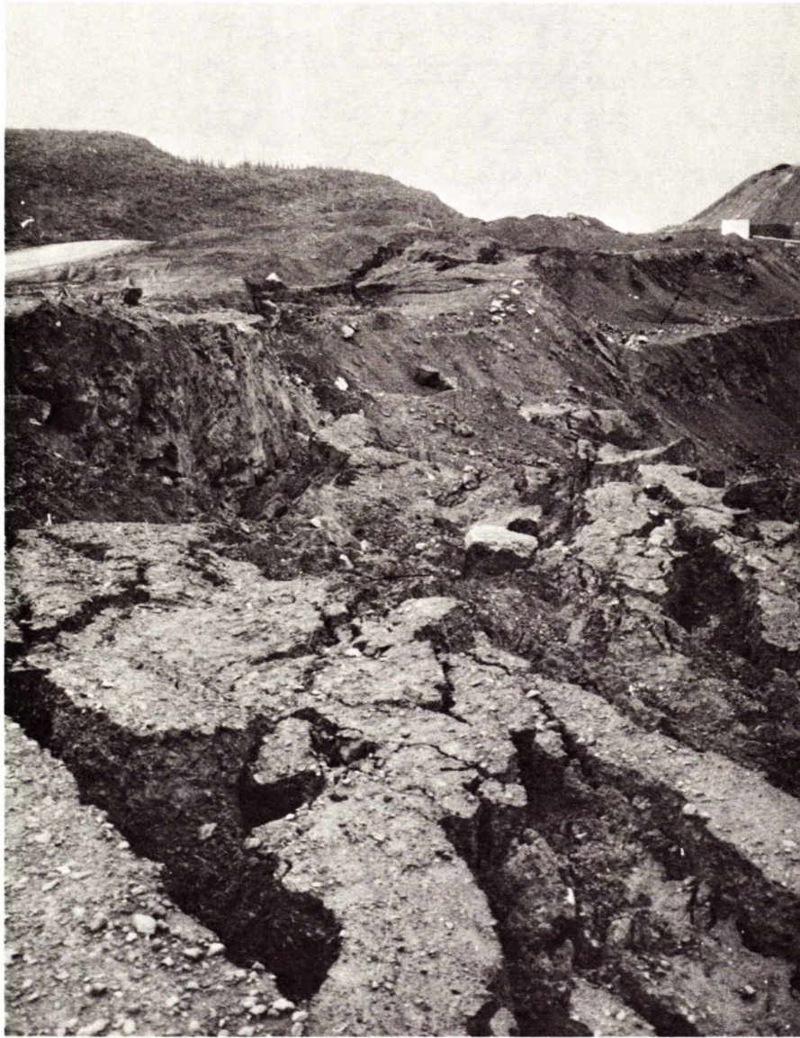
Figure 5. The continuing cracking in the same crest, September, 1962.
