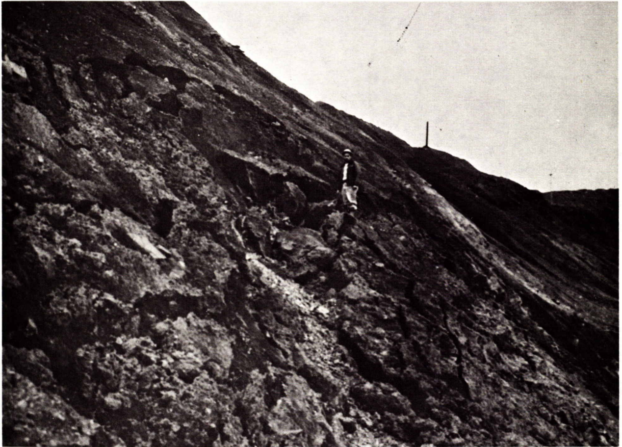
Figure 3. A small slide in the same wall, adjacent to the main slide zone, July, 1961.
