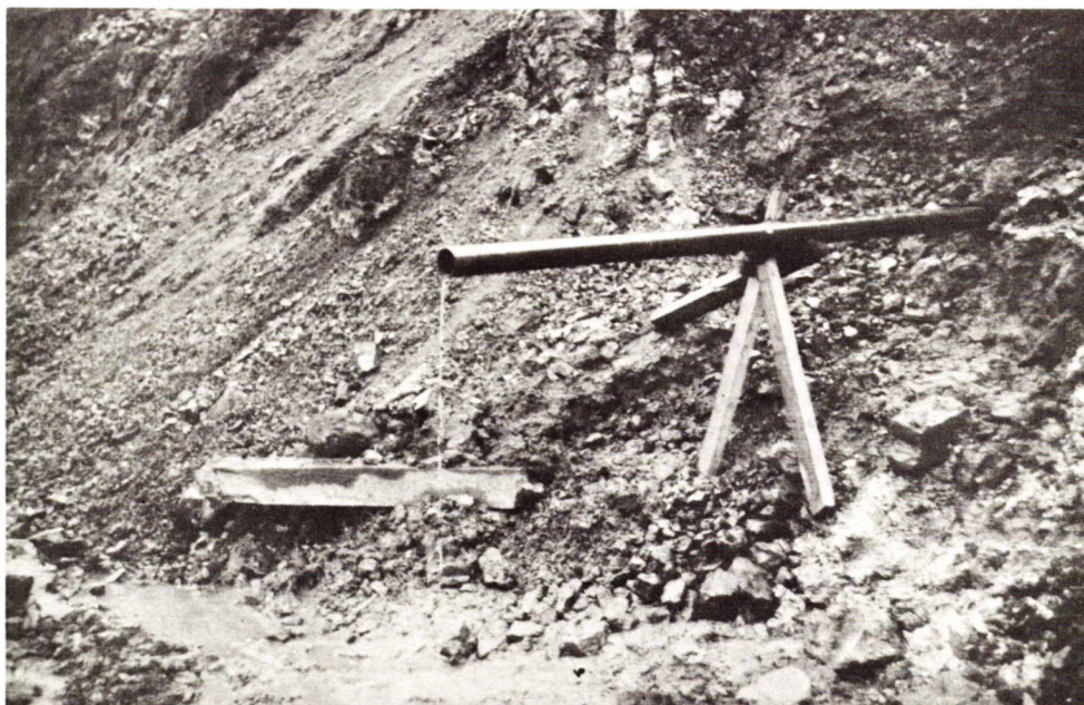
Figure 10. Horizontal drainpipe, July, 1963.
