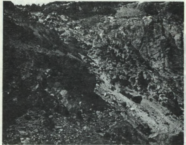
Fig. 14 - Slide No. 7 in ash rock.
