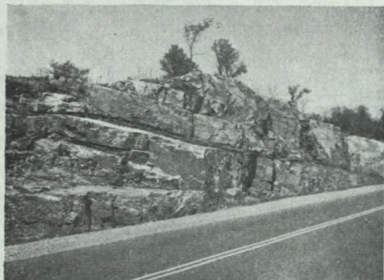
FIG. 3—Geological structures favouring plane shear failure.
