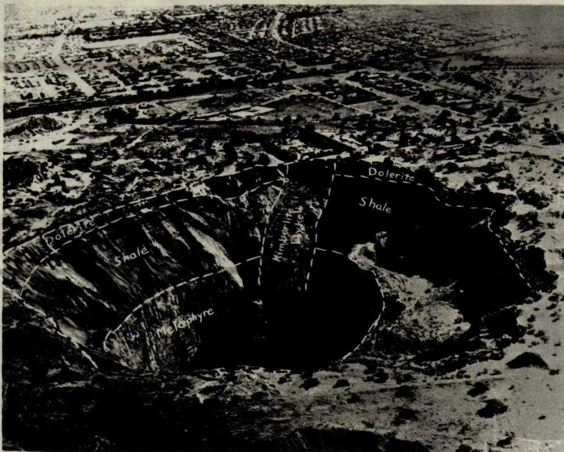
Photo 5. (ii). Oblique view of Bultfontein Mine big hole showing slopes (on the right side of the photo) which have broken back excessively due to abnormal ground water conditions and accordingly were not included in the analyses.
