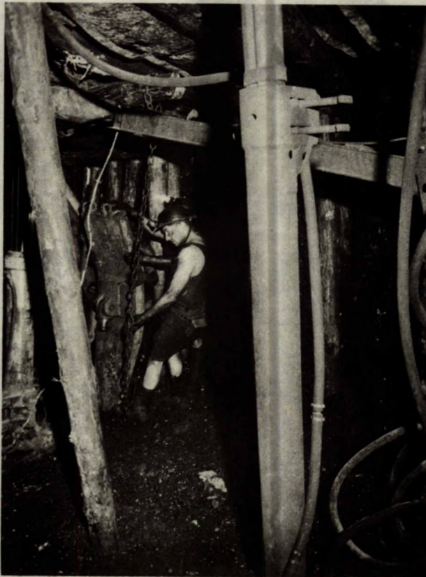
(g) ASSEMBLY OF THE BANANA PROPS.
