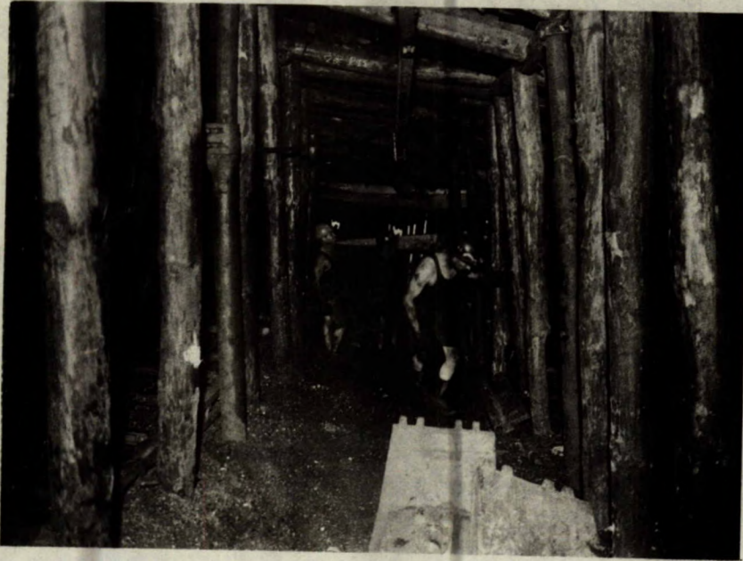
(f) TIMBER SUPPORTS ON THE FACE PRIOR TO THE INSTALLATION OF THE POWERED SUPPORTS; NOTE THE MONORAIL.
