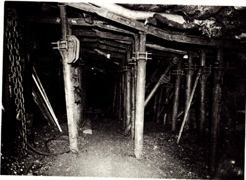
(e) AFTER REMOVAL OF THE POWERED SUPPORTS, THE FACE IS SUPPORTED BY THREE ROWS OF FRICTION PROPS.
