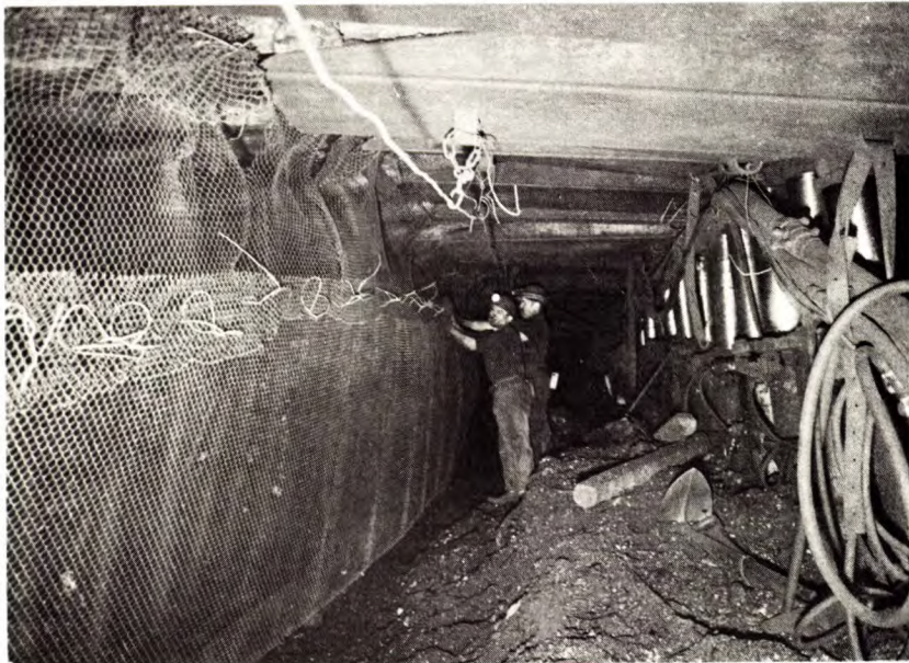
(e) Extending the mesh - Face D
