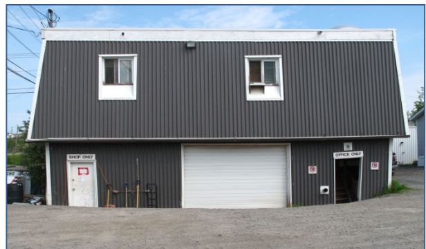
Ground subsidence related to warming of thaw-sensitive permafrost. NRCan contributes to the development of new codes and standards of building construction on permafrost. Photo by S. Wolfe.
