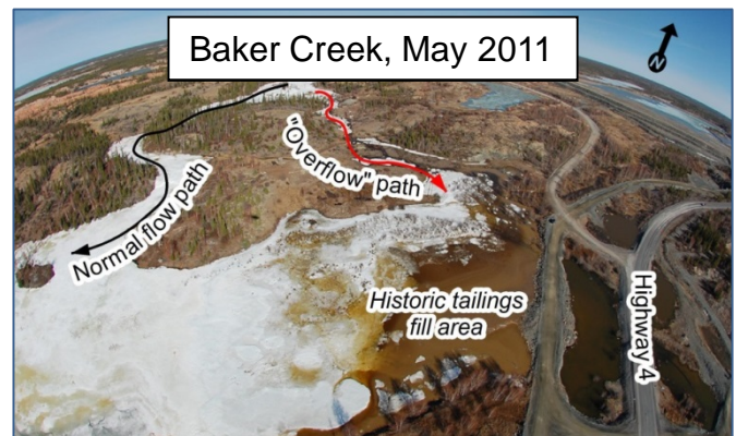
Winter icing formation on Baker Creek, near Yellowknife, NT, encroaching on adjacent tailings fill and highway embankment. Photo by P. Vecsie.
