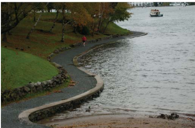
FIGURE 14: Hard armouring of the shoreline, Nova Scotia. Photo courtesy of M. Davies.
