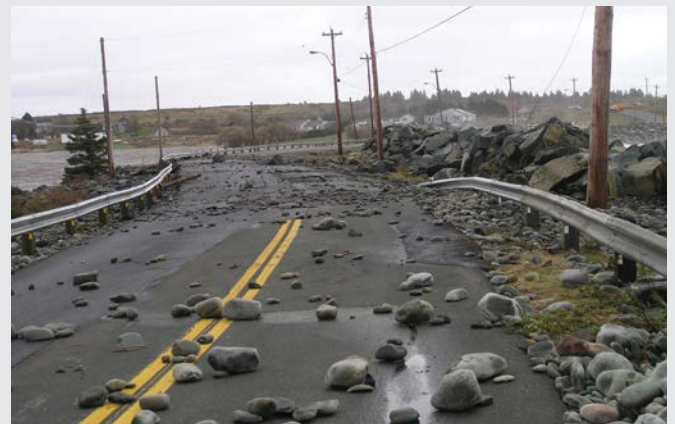
FIGURE 15: Effects of storm-wave overwash on Cow Bay Road, Halifax Regional Municipality, NS. Photo courtesy of R.B. Taylor.
