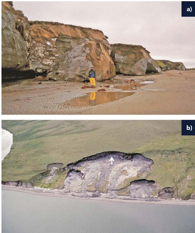
FIGURE 12: Erosion of permafrost coasts in the western Canadian Arctic: a) a deep thermoerosional niche undercutting cliff in ice-bonded sand and associated block failure following a major storm, Tuktoyaktuk Island, NT (Photo courtesy of S.M. Solomon, Natural Resources Canada, August 2000 ) and b) retrogressive thaw amphitheatres in ice-rich deposits at King Point, YT (edge of lagoon at left). Note massive ice (indicated by white arrow) in lower part of the main headwall, which is ~5 m high. Photo courtesy of D.L. Forbes, Natural Resources Canada, July 1992 .
