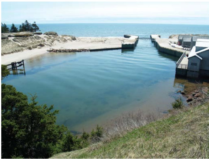
FIGURE 16: Hybrid protection at Basin Head, PE. Buried revetment covered with sand dune and marram grass. Photo courtesy of M. Davies.
