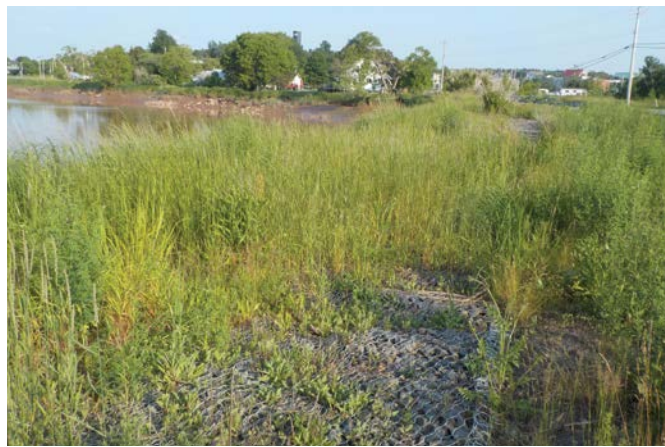
FIGURE 24: Hybrid living shoreline on the Shubenacadie River, Bay of Fundy, NS, illustrating gabion basket planted with marsh vegetation to reduce erosion scour. Photo courtesy of V. Leys, August 2015.
