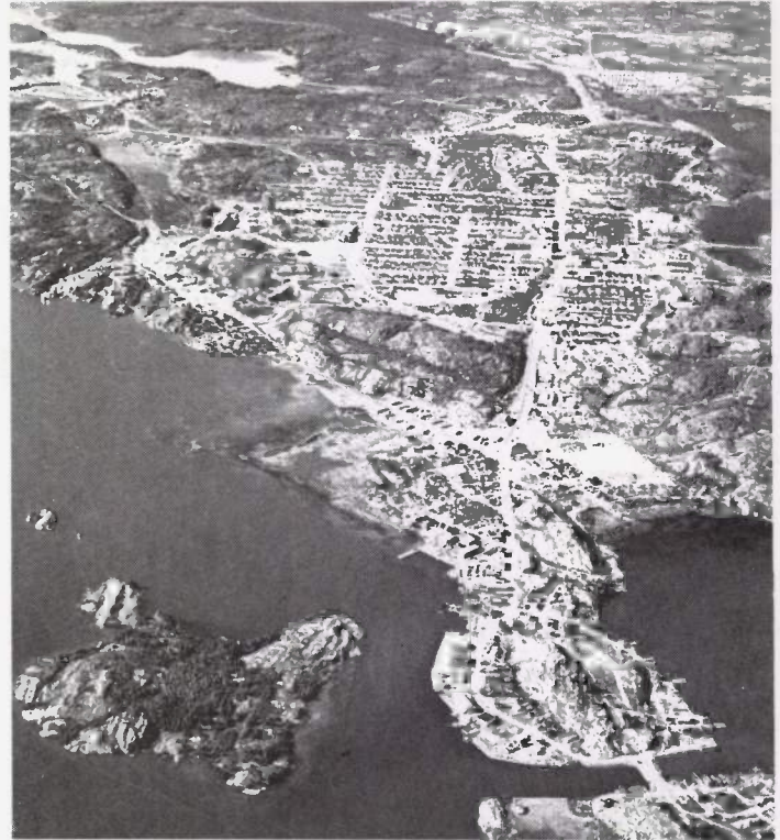
Aerial view of Jolliffe Island (bottom left) in the early 1970s. By this time the fuel tanks had been moved across Yellowknife Bay past Con Mine and almost all the houses had been moved from the island. The old and new town of Yellowknife can be seen in the centre of the photograph
