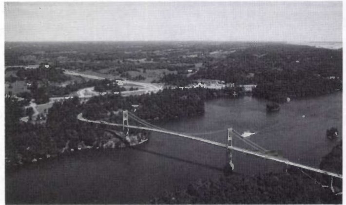
Part of the Thousand Islands Bridge linking Ontario with New York State. View looking east through the Raft Narrows within Canadian waters. Ivy Lea Provincial Park is on the left, and Georgina Island is in the right foreground; Surveyor Island can be seen at the entrance to Bucks Bay near the centre of the photo.
