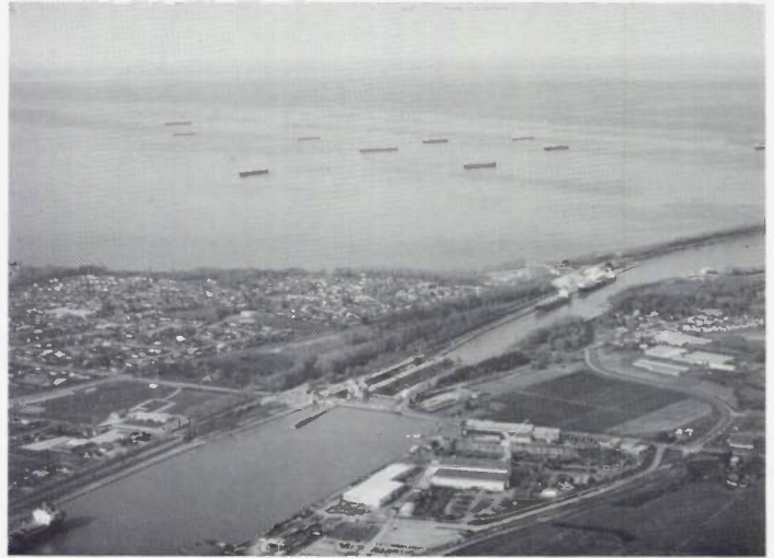
Northern entrance to the present Welland Canal at Port Weller. Lock 1, Bridge 1 and Port Weller Dry Dock are shown in the foreground
