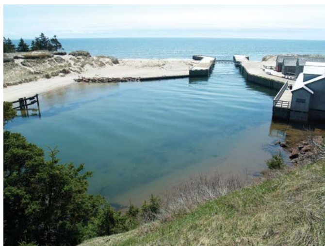
FIGURE 16: Hybrid protection at Basin Head, PE. Buried revetment covered with sand dune and marram grass. Photo courtesy of M. Davies.
