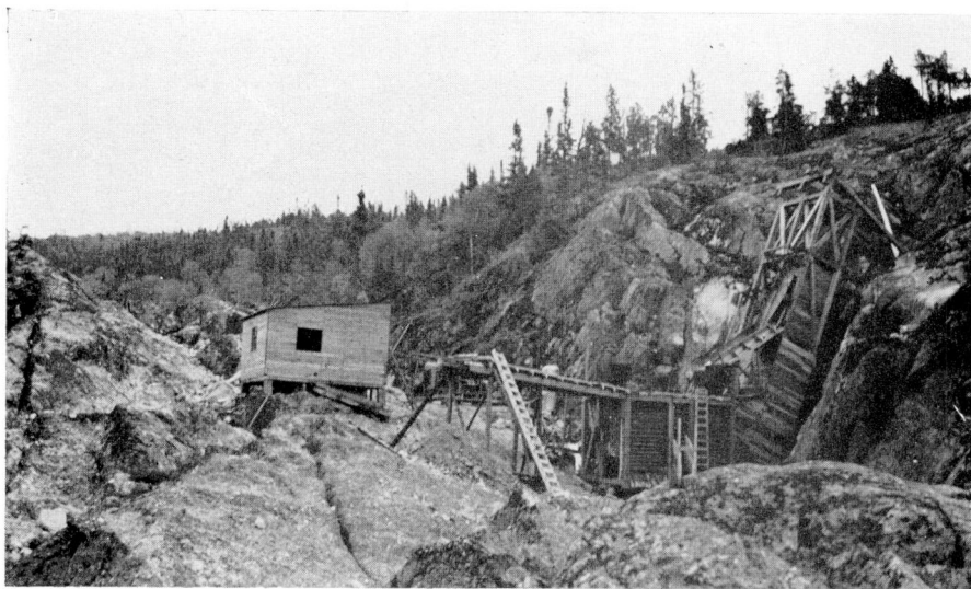
B. Inclined shaft on Camray property, Sault Ste. Marie region, Ontario. This shaft was begun in a depression formed by erosion along a diabase dyke. The shaft timbers were continued upward to form the headframe, which is anchored to the granite foot-wall of the dyke. (5-4, 1949.) (Page 125.)
