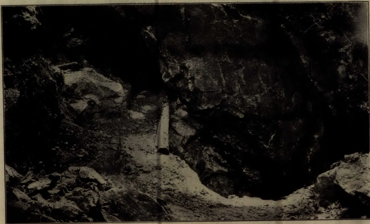
Drift and pit on inclined, pockety mica-apatite lead, range III, lot I, township of East Portland, Que. This illustrates the mode of occurrence and common method of working of the leads.
