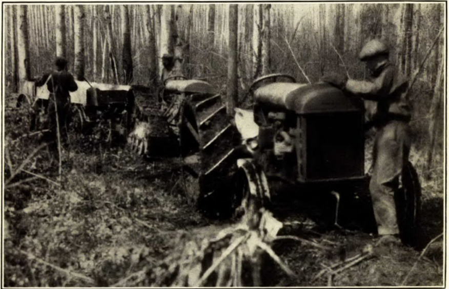
B. Tractors moving drilling equipment.
