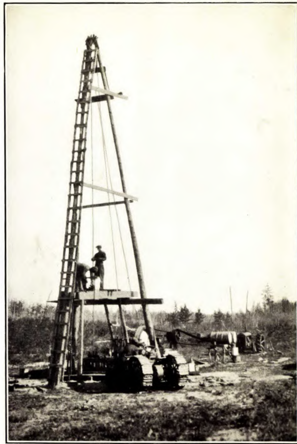
B. Drilling rig erected in sec. 25, tp. 93, R. 11. In foreground is a tractor used for handling drill rods, casing, etc. Another tractor belted to the draw-works is seen to the right of the derrick.
