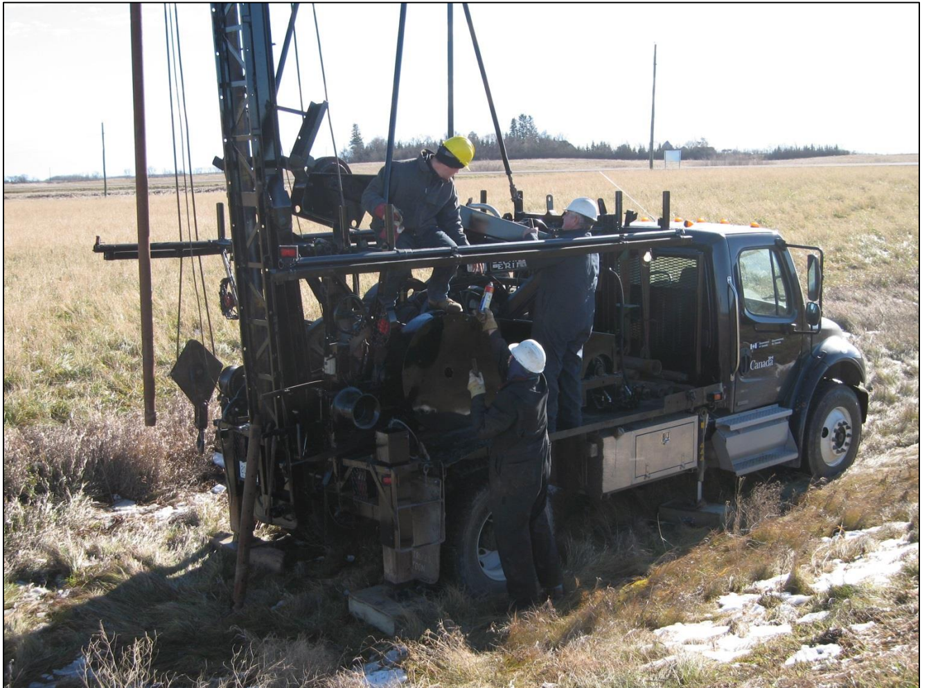
Photograph B1. AAFC B-12 drill rig setup with crew.
