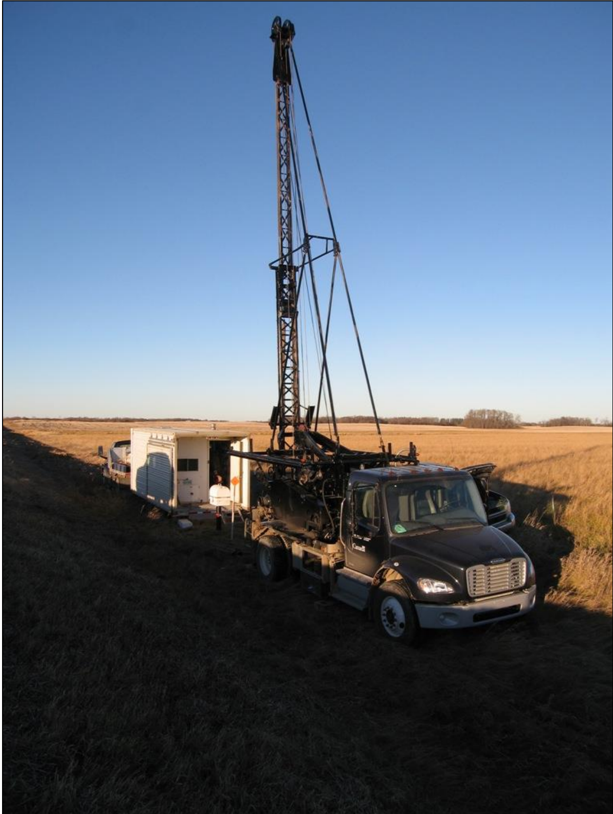
Figure 3. B-12 cable tool rig and field core logging trailer at site G05OA010 (GSC-BH-SW02), November 2010.
