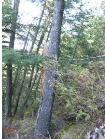
Figure 3. Tree being torn apart by spreading in hillside beneath its roots.
