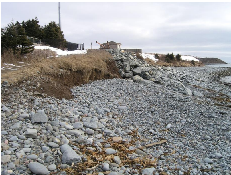
Figure 7. Cow Bay Beach: Armour rock at the eastern headland protects the immediate backshore but it accelerated adjoining bank erosion and interfered with the natural building of a pebble-cobble storm ridge similar to the one observed on both sides of the armour rock. The storm ridge was built as the February 9, 2013 storm waned.
