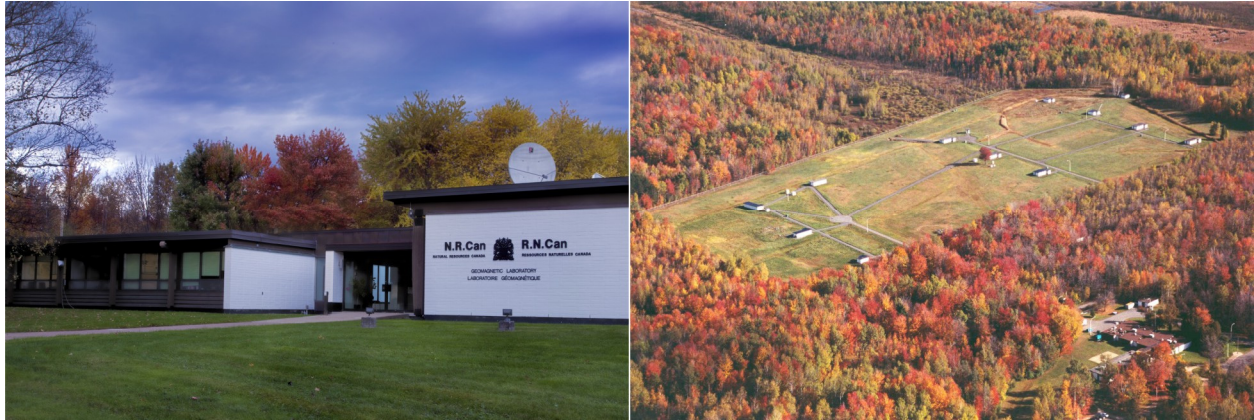
Figure 11: Images of the main building and compound for NRCan's Geomagnetic Laboratory.
