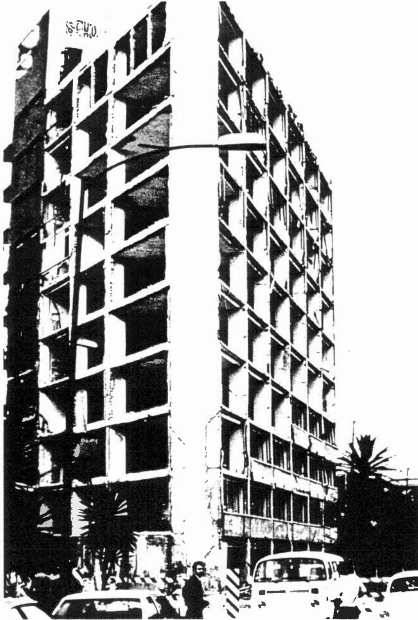
Fig. 6.6a Triangular-Shaped Reinforced Concrete Building
