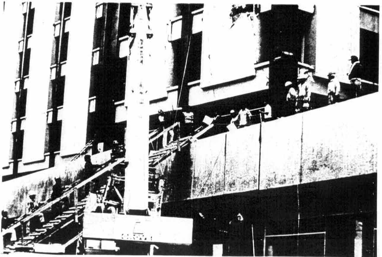
Fig. b.7d and b.7e Framing System and buckled corner column
