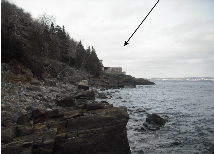
Fig. 30 a) York Shore Battery, from a distance.
