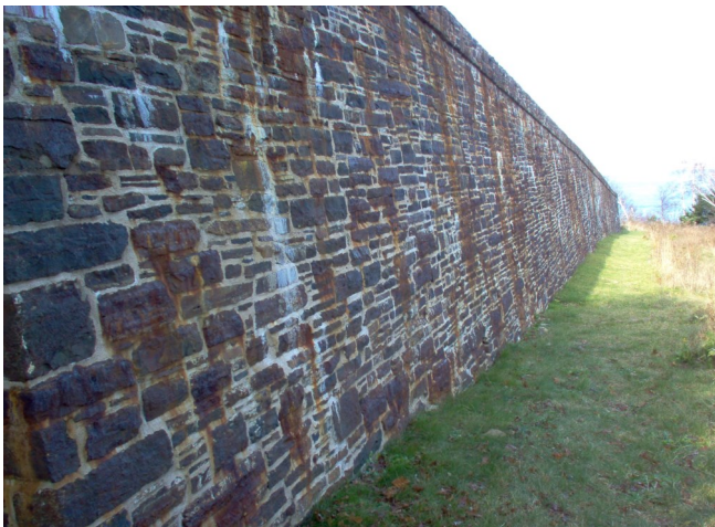
Figure 22. a) Base of wall at lower sally port entrance.
