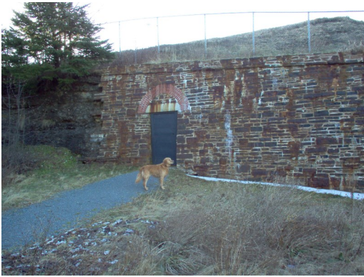
Figure 20. Sally port exit at base of wall
