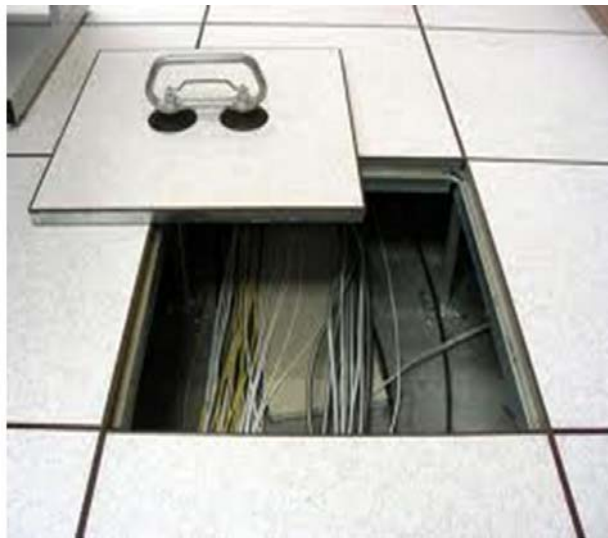
Figure 72: A typical raised floor system.
