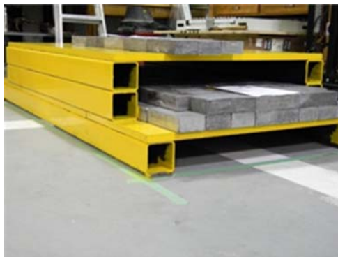
Second layer of lead in stalled.
