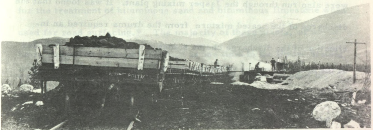
FIGURE 5. First trainload of bituminous sand for road surfacing at Jasper Park, Alberta.
