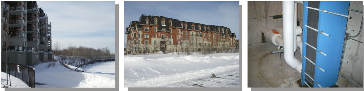
Figure 6.1. Images of the Goyer Quarry in Saint-Bruno-De Montarville, its condominium complex that uses surface water heat pumps, and the shared intermediate plate heat exchanger located in the building basement.
