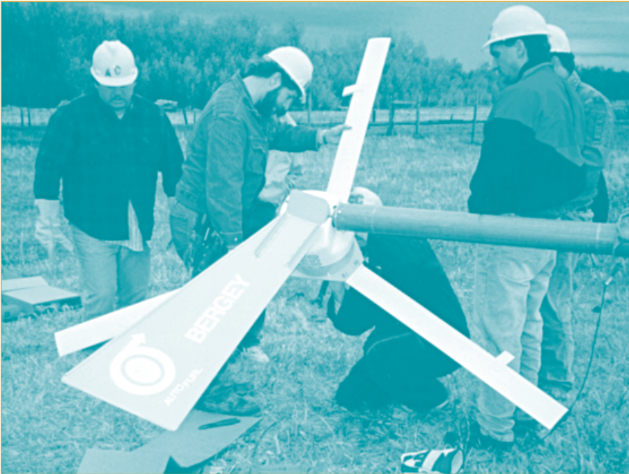
▲ Students of Assiniboine College in Manitoba install an 850 watt turbine. (Photo courtesy of Nor'wester Energy Systems Ltd.)
