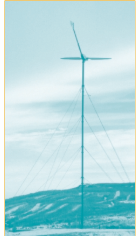
▲ Figure 9. A small 25kW Wenvor-Vergnet wind energy system in Collingwood, Ontario, supplies electricity to a rural residence. (Photo courtesy of Wenvor Technologies Inc.)
