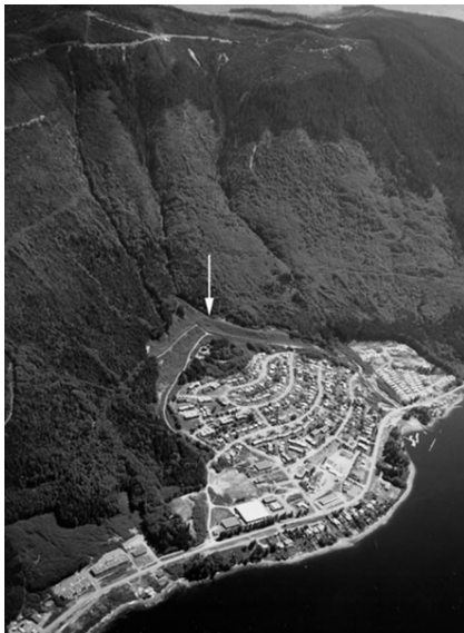
Figure 24. Debris Deflection Dykes. Debris deflection dykes (arrow), constructed in 1976, protect the town of Port Alice, Vancouver Island, from debris flows.
