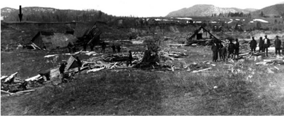
Figure 19. Notre-Dame-de-la-Salette landslide, Quebec. Contemporary photograph of destruction at Notre-Dame-de-la-Salette, western Quebec, showing effects of landslide-generated wave on wooden buildings located on east bank of Lièvre River in April 1908. Arrow indicates scarp of landslide on west bank of river.
