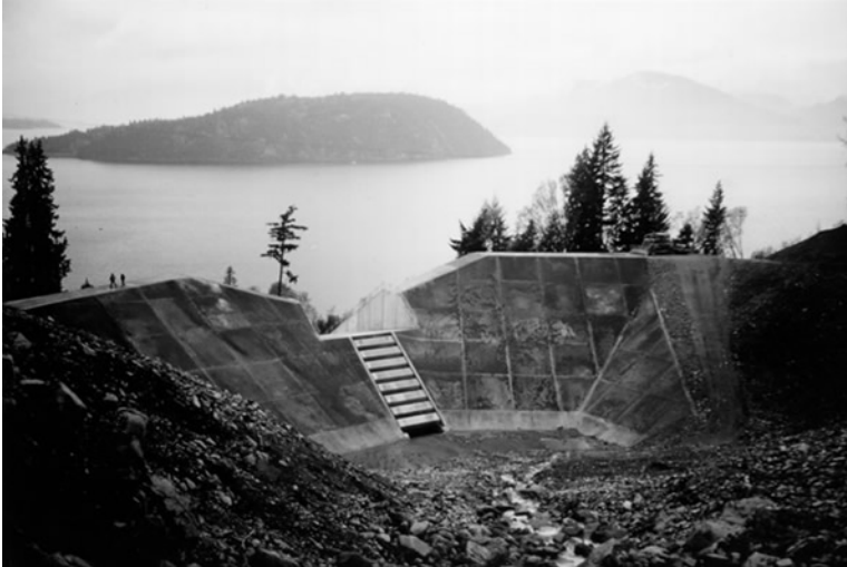
Figure 25. Catchment Dam. View down a debris flow pathway along Charles Creek, on Howe Sound, British Columbia, to a debris flow retention structure constructed in the mid-1980s to protect homes in Strachan Creek. The structure was designed to retain a debris flow event of 29 000 cubic metres.
