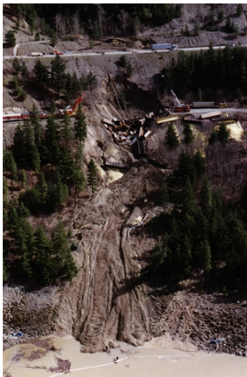
Figure 17. Railway Embankment Failure. Aerial view of a railway embankment failure which occurred at Conrad Siding, near Lytton, in the Fraser Canyon of southern British Columbia, March 1997. A freight train plunged into the pit caused by the failure, resulting in the death of two crewmen. The failure also undermined the Trans-Canada Highway, visible at the top of the photograph. The saturated fill material formed an earthflow which flowed down to the Fraser River in the foreground.
