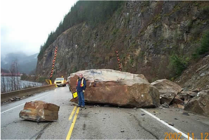
Figure 2. Rockfall on Trans-Canada Highway. Rockfall on Trans-Canada Highway, near Yale, British Columbia, triggered by heavy rains on November 9, 1990
