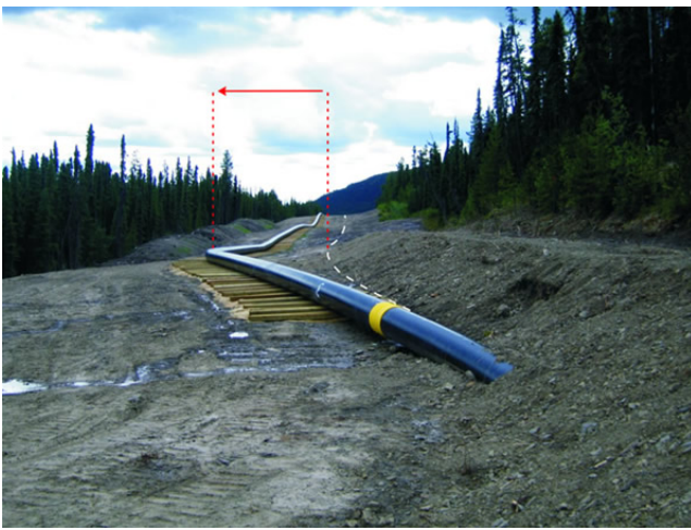
Figure 4. Creep. The slow downslope movement of erosional debris has displaced (arrow) a gas pipeline in northern British Columbia. Original position of pipeline is indicated by white dashed line. The pipeline has been placed on timbers to allow adjustment to continuing slope movement.
