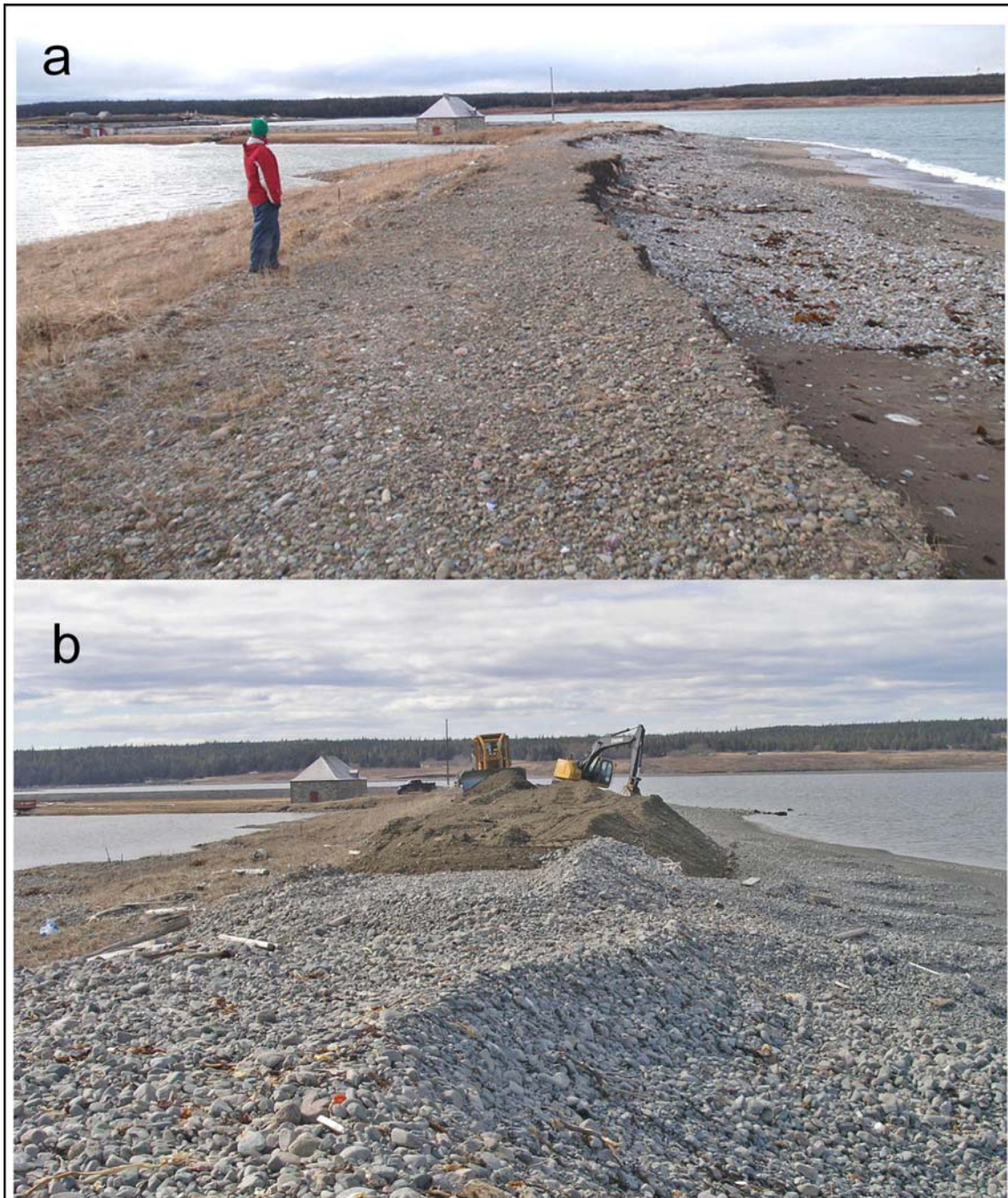
Figure 1541-3. Grand Étang Beach looking north (a) in January 2011 showing the narrow extent of upper beach that survived the four December 2010 storms (photo R. Duggan); (b) 31 March 2011 showing the beach crest rebuilding and seaward slope smoothing program . (b) also illustrates the significant difference in the composition of the new fill and the natural cobble beach (foreground) at the south end of the barrier beach. Pièce de la Grave Guardhouse in the background.
