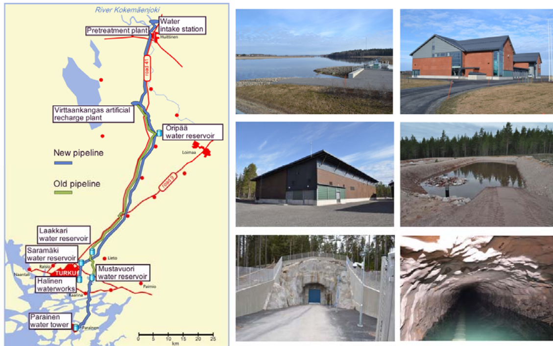
Figure 1. Managed aquifer recharge system of the Turku region - Location map and photos of the facilities.
