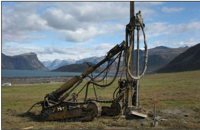
Figure 4: Deep drilling with the airtrack drill.
