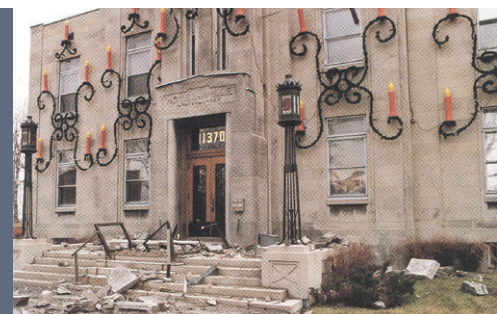
Former Montreal-East City Hall suffered damage to the masonry cladding, 1988.
