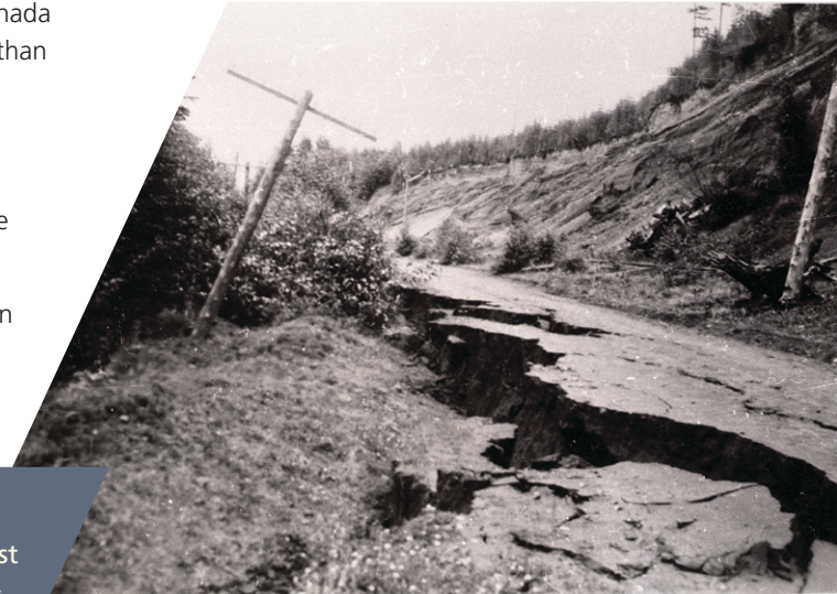
Road damage north of Campbell River, BC from the 1946 Earthquake.
