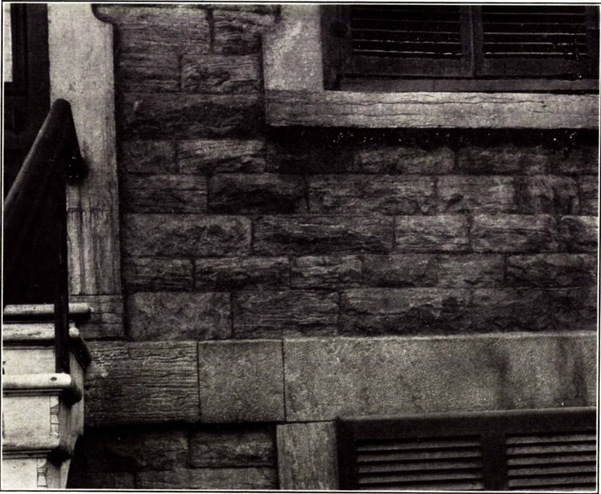
Montreal limestone. Building in Montreal showing the effect of weathering.
