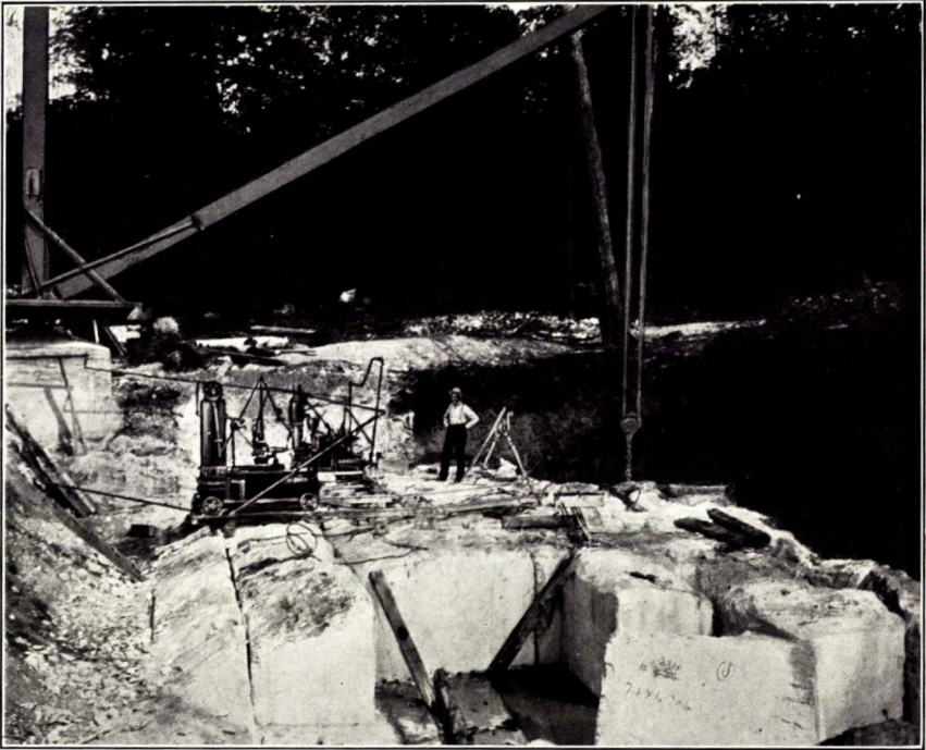
South Stukely marble. Cutting marble blocks from surface at the quarry of the Dominion Marble Company, South Stukely, Que.
