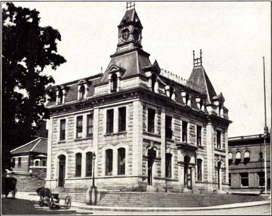
Stanstead granite. Post-office, Sherbrooke, Que.
