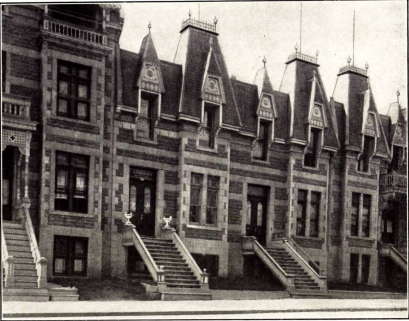
Montreal limestone. Buildings in Montreal showing the contrast between rock face and bush hammered work.
