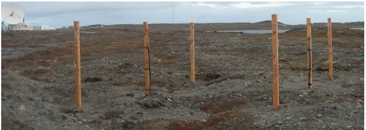
Figure 7. Riometer antenna support for dig-able ground conditions
