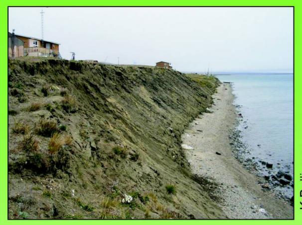
Eroding bluffs near Sachs Harbour
