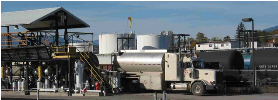
Figure 29. Rail terminal for petroleum products, Terrace. Gasoline and diesel brought in by rail car is stored and transferred to tanker trucks for distribution to gas stations.
