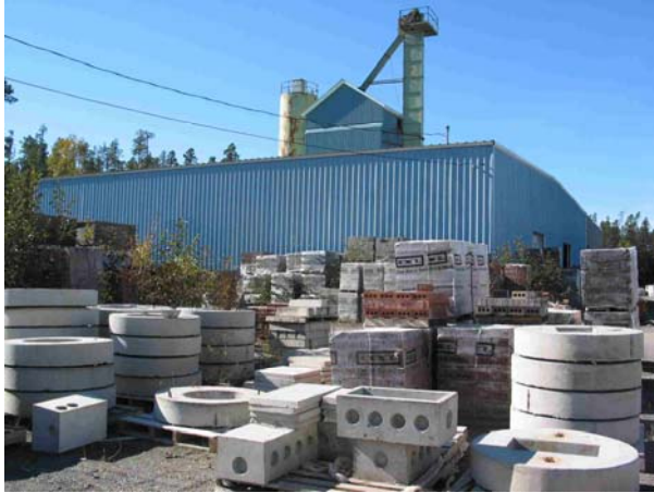
Figure 27. Concrete plant on Old Lakelse Lake Drive in Thornhill. The plant makes concrete aggregates, septic tanks, highway barriers, brick, block, paving stones, slabs, chimney blocks, and premixed sack products.
