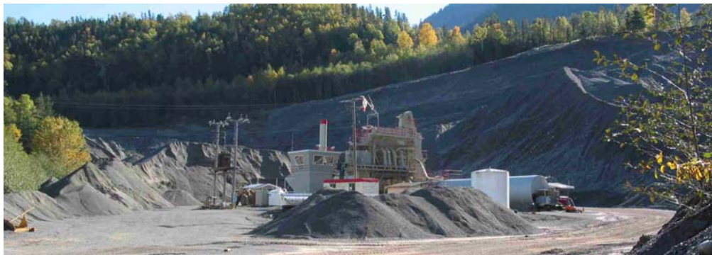
Figure 28. Asphalt plant on along Highway 16 east of Thornhill. Sand and gravel are quarried from Ice Age deposits, sorted, and combined with liquid asphalt at the plant.
