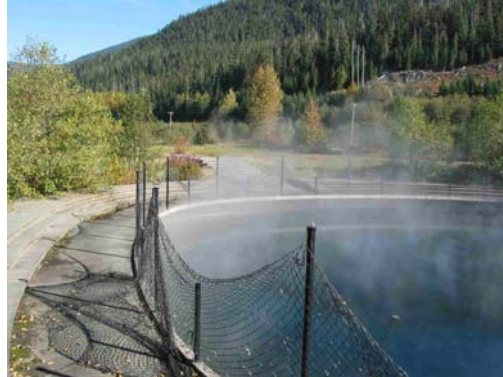
Figure 21 and 22. (left) Swimming pool at hot springs. (right) Unused concrete pool built around one of the hot springs. Photos by Bob Turner. Mount Layton hot springs, also known as Lakelse hot springs, include at least half a dozen warm seeps that straddle Highway 37 and flow into wetlands that surround the resort area. Warm springs may also occur on the floor of Lakelse Lake, as soft spots are reported in the winter lake ice by locals.
