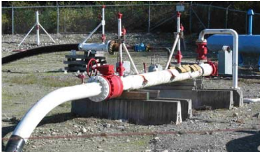
Figure 29. Rail terminal for petroleum products, Terrace. Gasoline and diesel brought in by rail car is stored and transferred to tanker trucks for distribution to gas stations.
