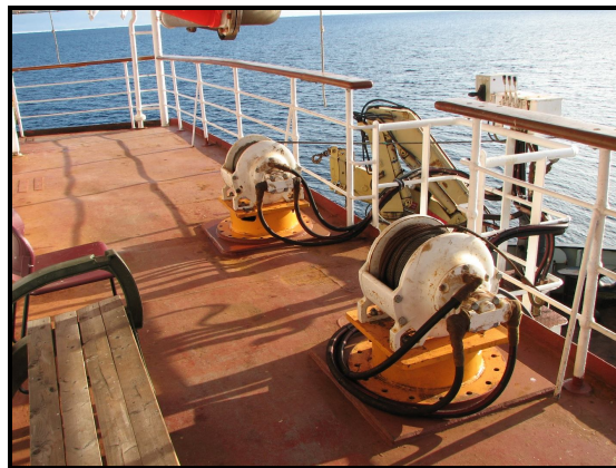
Figure 5.5 Two recovery tugger winches fitted to the tween deck; also note the hydraulic control station for these winches and the ship's A frame controls.
