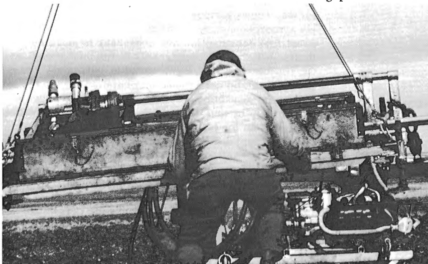
Figure 5. Positioning the platform and mast.
