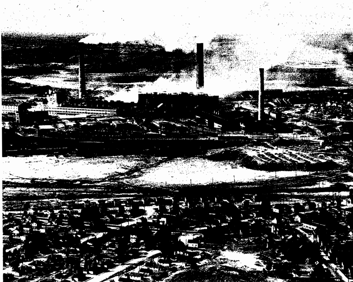
Located at Copper Cliff, Ontario, International Nickel Company's mill has a capacity of 30,000 tons of ore a day. The smelter has seven reverberatory furnaces and nineteen converters.
