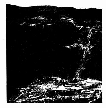
In south-central British Columbia, Craigmont Mines Limited began production from its copper mine. Ore from the open pit on the mountain slope (top) is trucked to a primary crusher and then carried on a one-mile cable belt to the mill and concentrator below (left). Concentrates are shipped to Japan and the United States.
