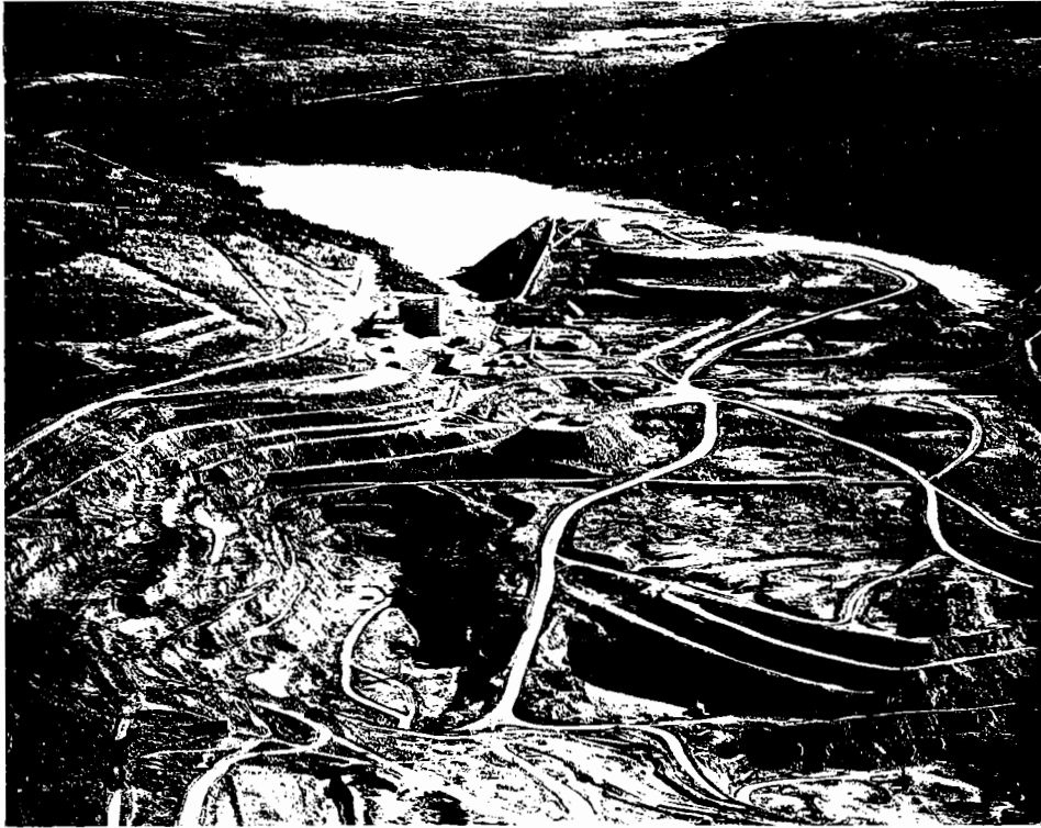
The open pit and mill of Lake Asbestos of Quebec Ltd. at Black Lake in the Eastern Townships of Quebec. In order to expose the orebody, which was under Black Lake, extensive dredging and draining had to be done. The remnants of the lake can be seen in the background. The Eastern Townships produce most of Canada's asbestos and 40 per cent of the world supply.
