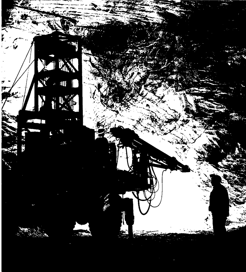
Drill jumbos are used to drill off the salt face.
