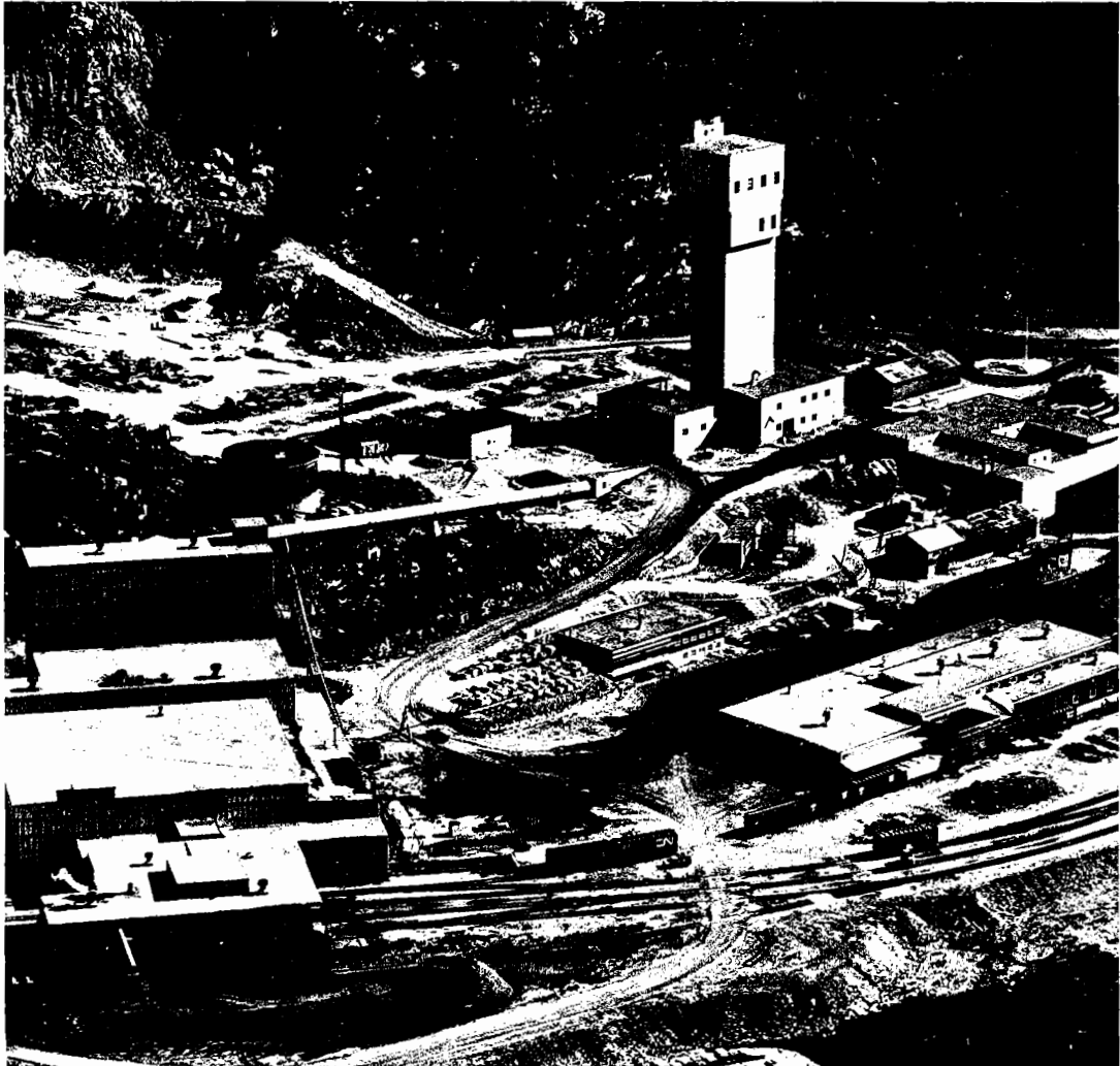
Geco Mines Ltd., Manitouwadge area. Mill and service buildings and principal head-frame.
