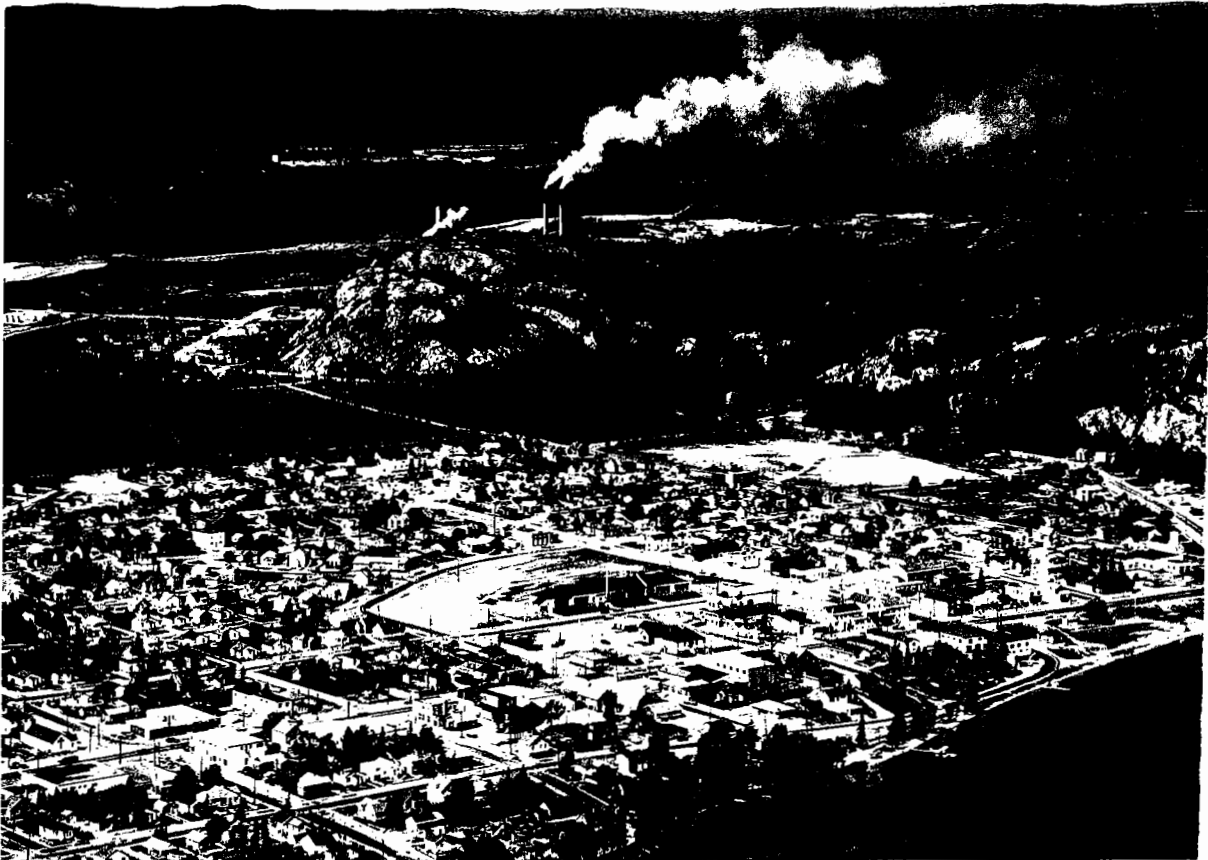
The Algoma Steel Corp. Ltd., Wawa, with treatment plant in background.
