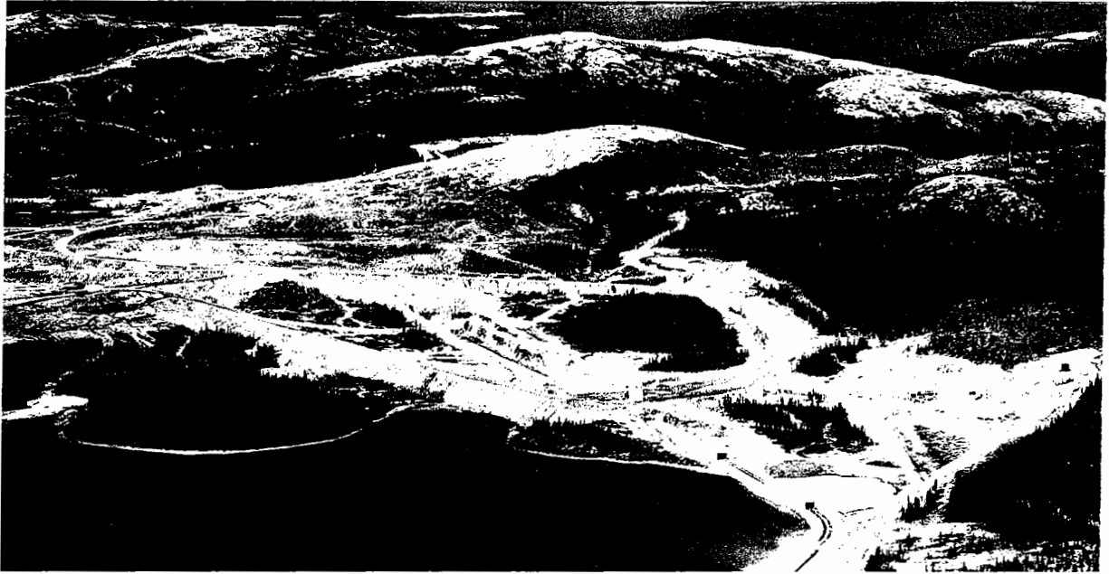
Iron Ore Co. of Canada, over-all aerial view of the Carol Lake orebodies.
