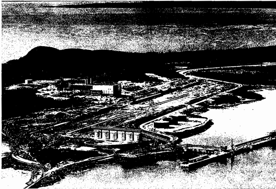
Aerial view of Pointe Noire harbour, storage silos and plant under construction.
