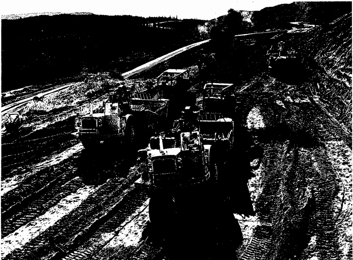
Stripping operations at the Endako mine.
