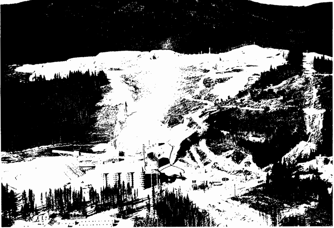
The molybdenum operation of Endako Mines Limited in central British Columbia, shortly after it began operations in June 1965.
