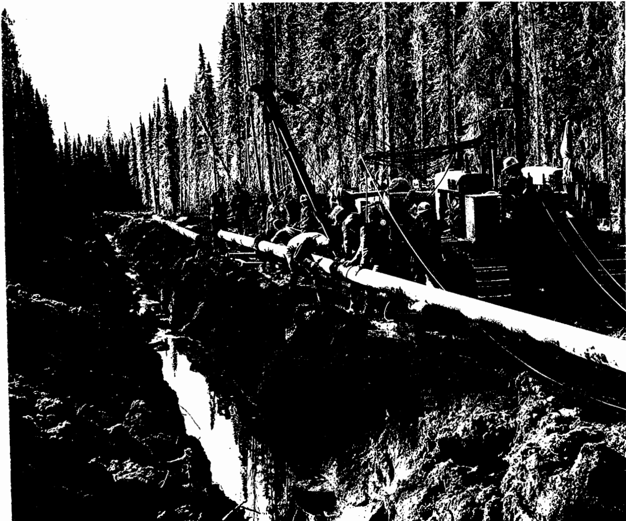
Installation of a natural gas gathering line in Alberta.
