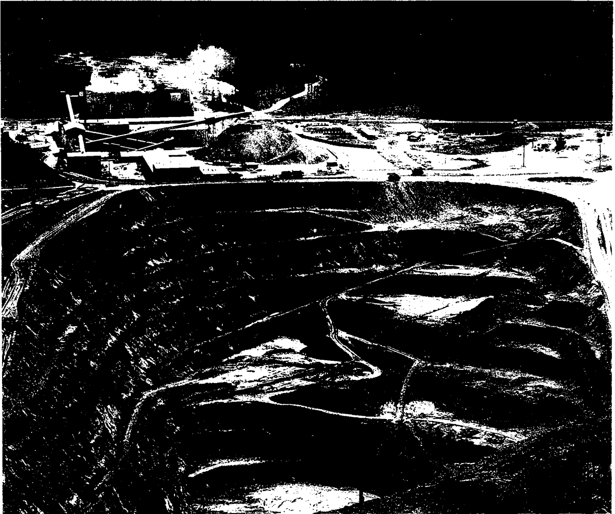
The benches in Placer Development Limited's Endako open-pit mine in northern British Columbia form a sharply defined pattern, with the mine concentrator in the background. The mine is a molybdenum producer. (George Hunter photo).
