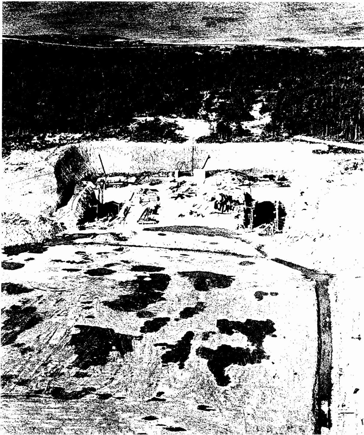
Core drilling offshore north of Cape Perce and Donkin village on Cape Breton Island, Nova Scotia, outlined a huge undersea coal reserve of 1.8 billion tonnes. The Cape Breton Development Corporation (DEVCO) was authorized to tunnel out to a point where mining can begin and work on the twin tunnels as shown here, with the ocean in the background. (Gordon photo, courtesy DEVCO)
