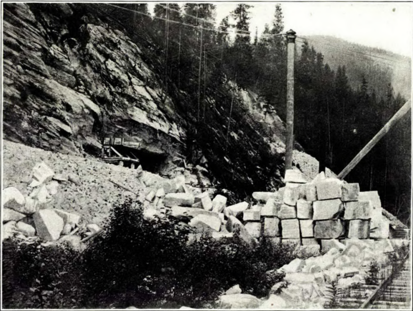
Marble blocks and portal of quarry of the Canadian Marble and Granite Works, Marblehead, B.C.
