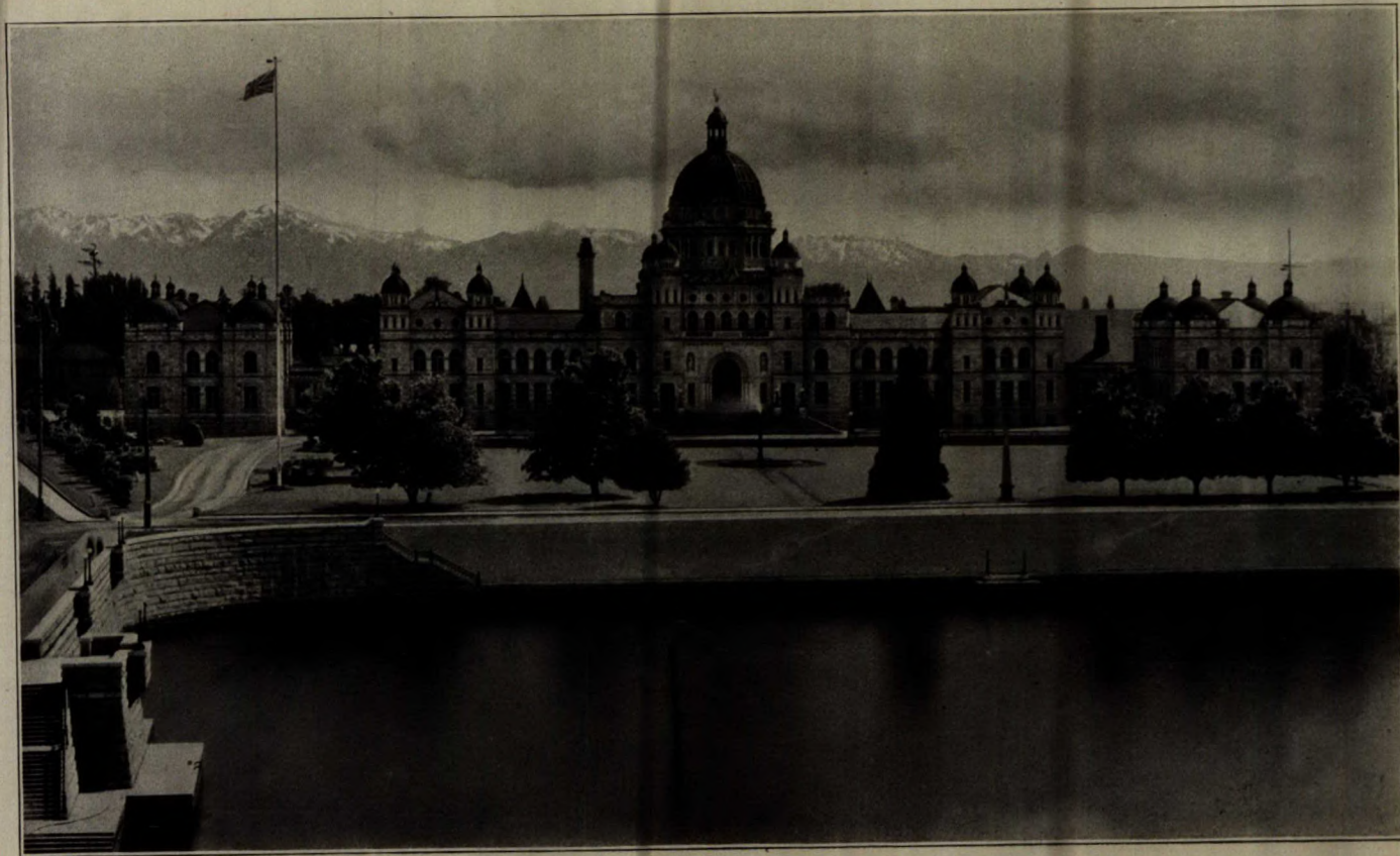
Haddington Island andesite and Jervis Inlet granite. Buildings of the Legislative Assembly of British Columbia, and sea-wall, Victoria, B.C.
