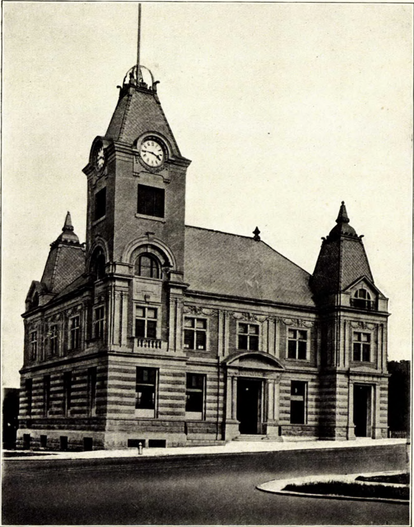
Mayne Island sandstone. Post-office at corner of Main and 15th streets, Vancouver, B.C.
