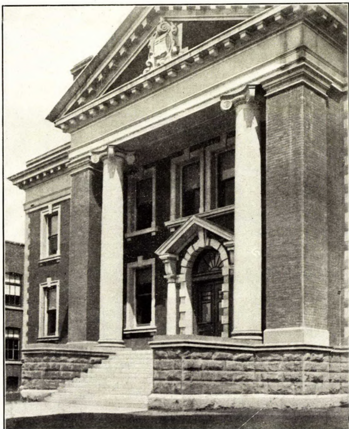
Paskapoo sandstone, Macleod Quarrying and Contracting Company's quarry. Court house, Lethbridge, Alberta.
