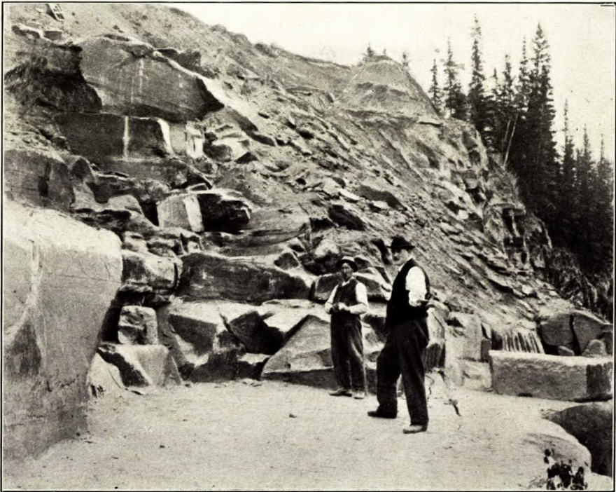
Paskapoo sandstone. Upper beds in quarries of Pembina Quarries, Limited, Entwistle, Alberta.
