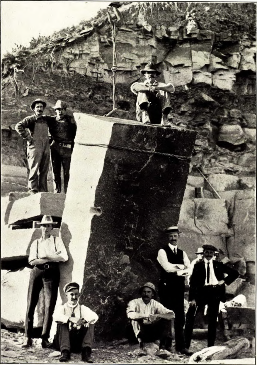
Paskapoo sandstone. Lifting a block in the quarry of the Macleod Quarrying and Contracting Company, Monarch, Alberta.
