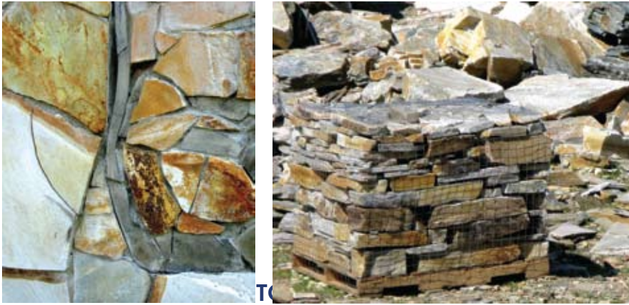
Figure 81. (Left) Close-up of quartzite in stone murals. Natural iron oxide pigments stain the white quartzite rock a variety of colours.
