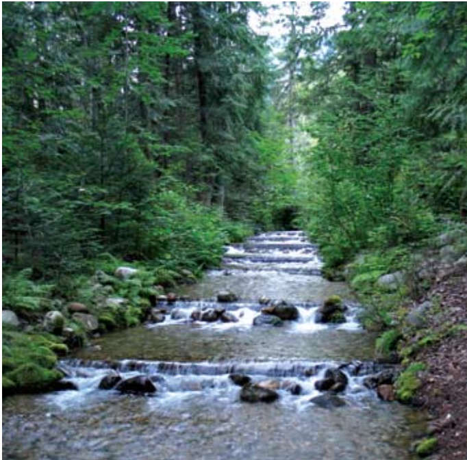
Figure 22. (Left) This spawning channel has been constructed by fisheries engineers within an abandoned side channel of Kokanee Creek. Engineers use a particular size of gravel that is small enough for kokanee salmon to dig nests, but large enough for eggs to fit in the spaces between pebbles. A staircase of falls and pools encourages circulation of stream waters into the stream bed and back to the stream, carrying oxygen and nutrients to the eggs within the gravels. (Top Right) Kokanee salmon return each autumn to Kokanee Creek to lay eggs in the stream gravels (photo courtesy of BC Parks). (Lower right) Kokanee eggs in stream gravels (photo courtesy of BC Parks). The eggs live within stream gravels through the winter. Young salmon hatch in the spring and continue to live within the gravels until they are ready to emerge.
