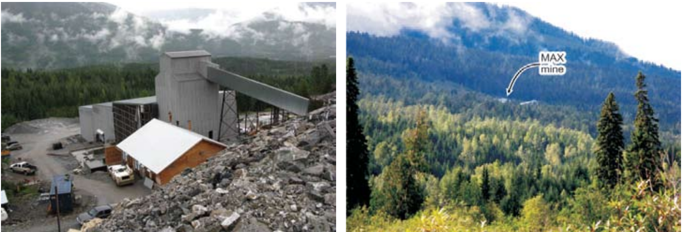
Figure 62. (Left) The mill at the MAX mine. (Right) MAX mine buildings viewed from the valley floor near Trout Lake.
