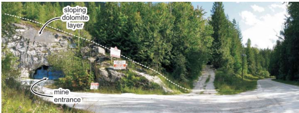
Figure 34. The entrance to the underground dolomite mine is at a former quarry on Crawford Bay Road. The blue doors control access to the mine tunnel. The quarry cliffs above the door are pale-coloured dolomite. Prior to underground mining, the dolomite was extracted from the surface quarry. The golf course is across Crawford Bay Road to the right.
