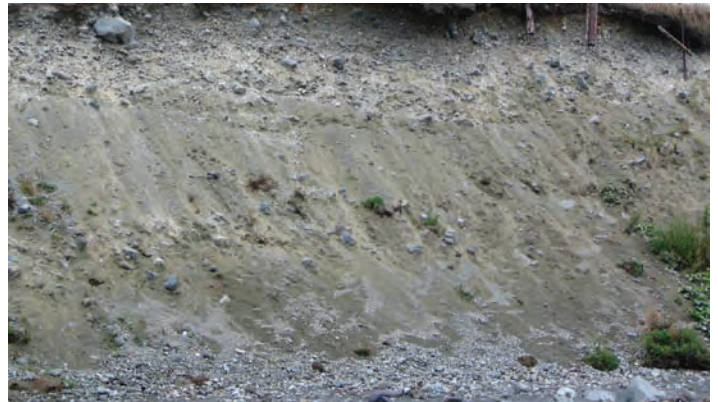
FIGURE 14: a) Coastal erosion, Union Corner Provincial Park, PE and b) Active bluff erosion, Middle Cove, NL.
