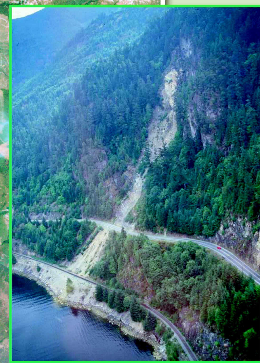
Photograph of rockslide at Loggers Creek, October 1990, taken by O. Hungr. Damage was estimated at > $7M when a large rockslide closed the highway and rail line for 13 days.
